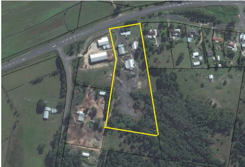
Figure 4: Aerial Photo of Surrounding Environment (source: Clarence Valley Council GIS)
